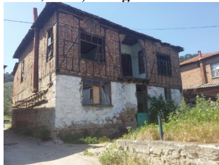
Figure 5. Mixed system (Tuztaş, Çobancaoğlu, 2006)
