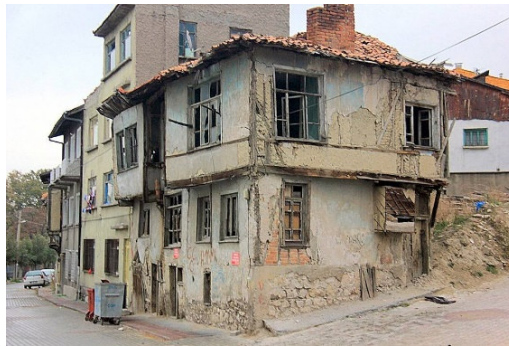
Figure 6. Traditional house with adobe infilled system in Kütahya (Şaşmaz, 2019)
