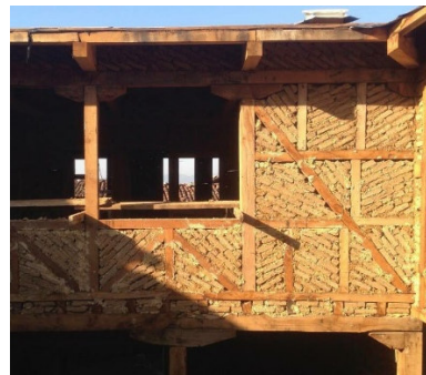
Figure 4. Adobe infilled system (Bilgili, 2018)
